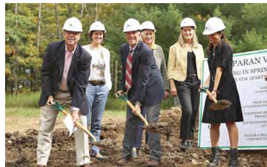
▲ Governor Scott joined the ground breaking for Lake Paran Village in Shaftsbury, where Shires Housing is developing 22 new apartments.
